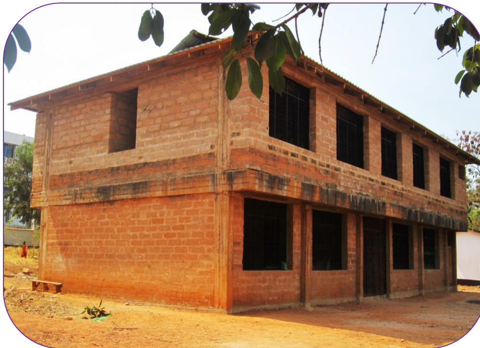
National Bureau of Statistics' building in Kigoma as recently captured by our photographer during Dr. Chuwa visit in Kigoma
