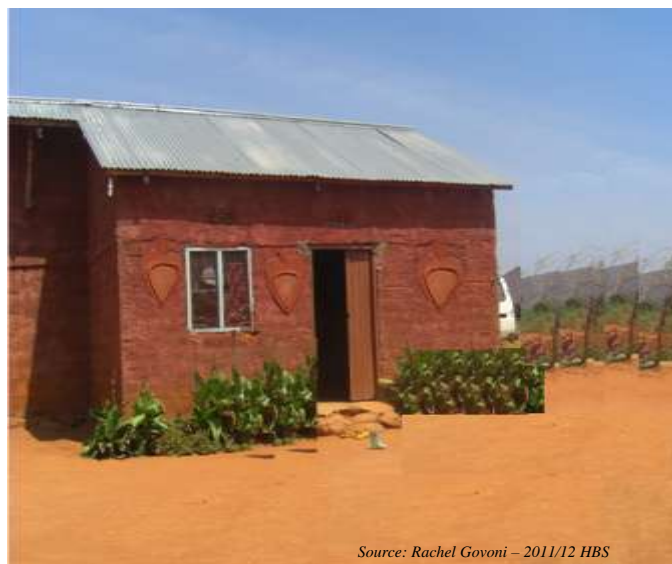
Picture No. 1: A building with Burnt Bricks and Iron Sheets
