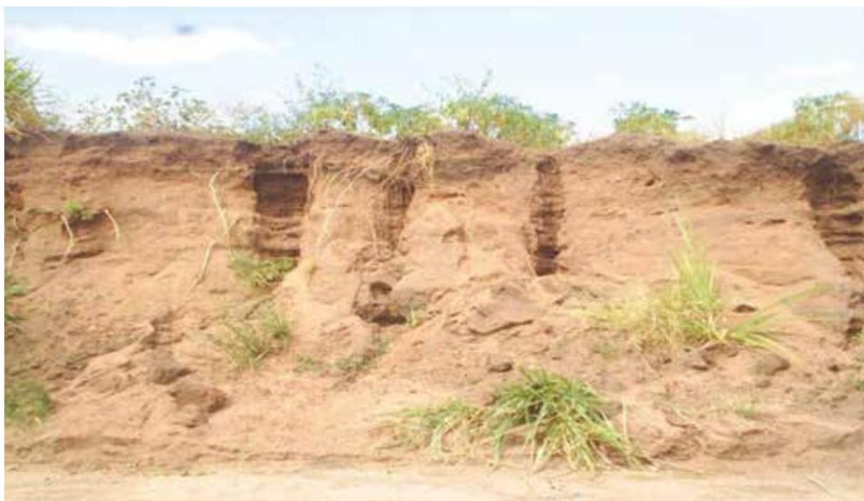
Figure 3. 2: Evidence of severe gully erosion in Bunda district
