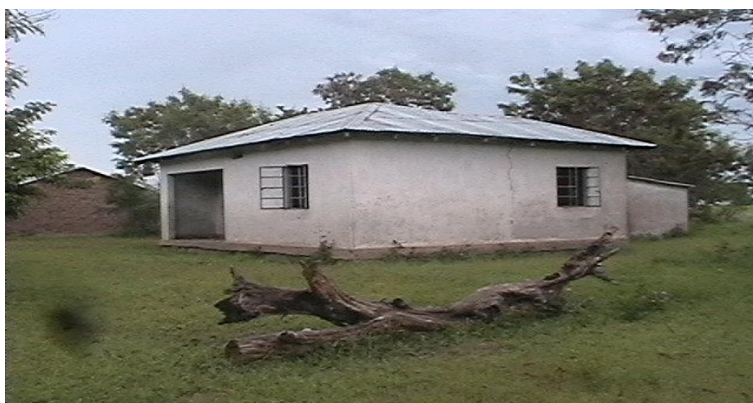
The use of metal roofing and cement block walls are most common in urban areas.
